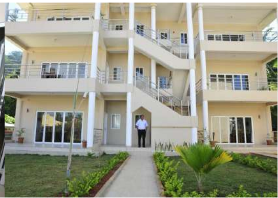
Exterior View of Apartments
