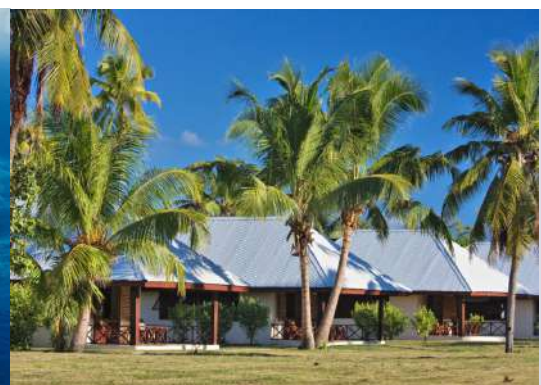
Exterior View of Villas
